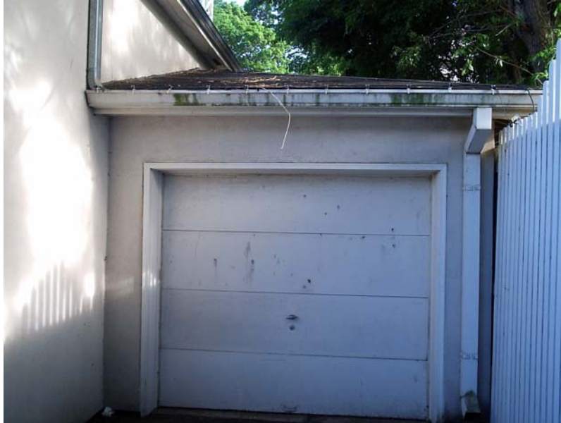
Pre-treatment exterior surfaces on a residence.
