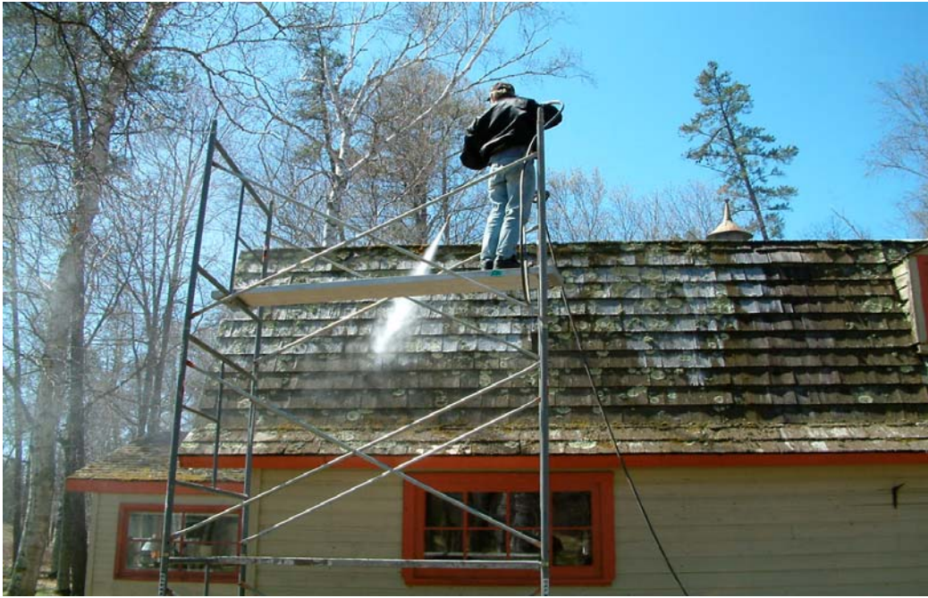
Heavily contaminated roofs can be effectively treated with MDF Roof Pro.
