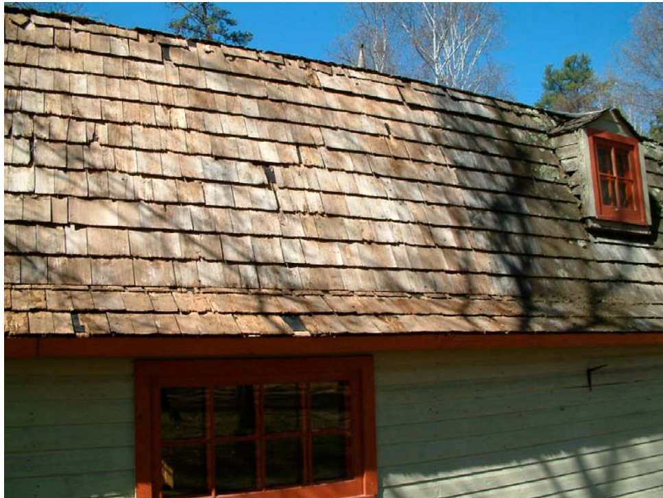
Post-treatment with MDF Roof Pro
