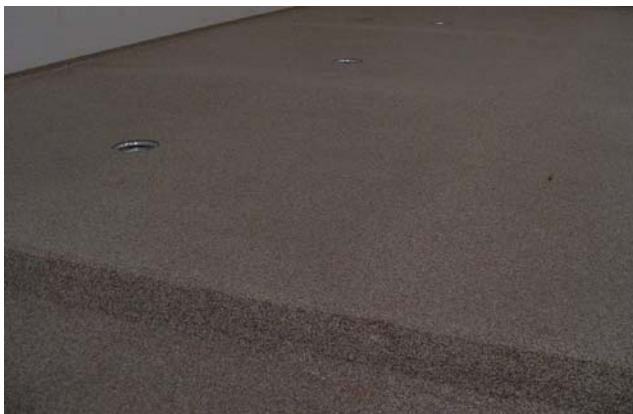
Individual shower stalls are sloped to drains to prevent cross contamination between shower stalls.
